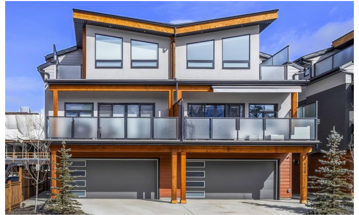
UNIT 1 AT 826 7TH STREET IN CANMORE ALBERTA
